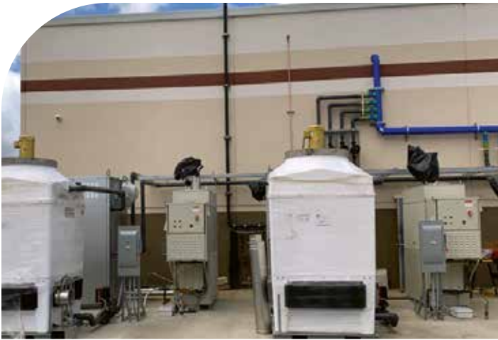
Six Capstone C65 microturbines help Leaf California meet their sustainability goals on improved energy efficiency while reducing waste.
